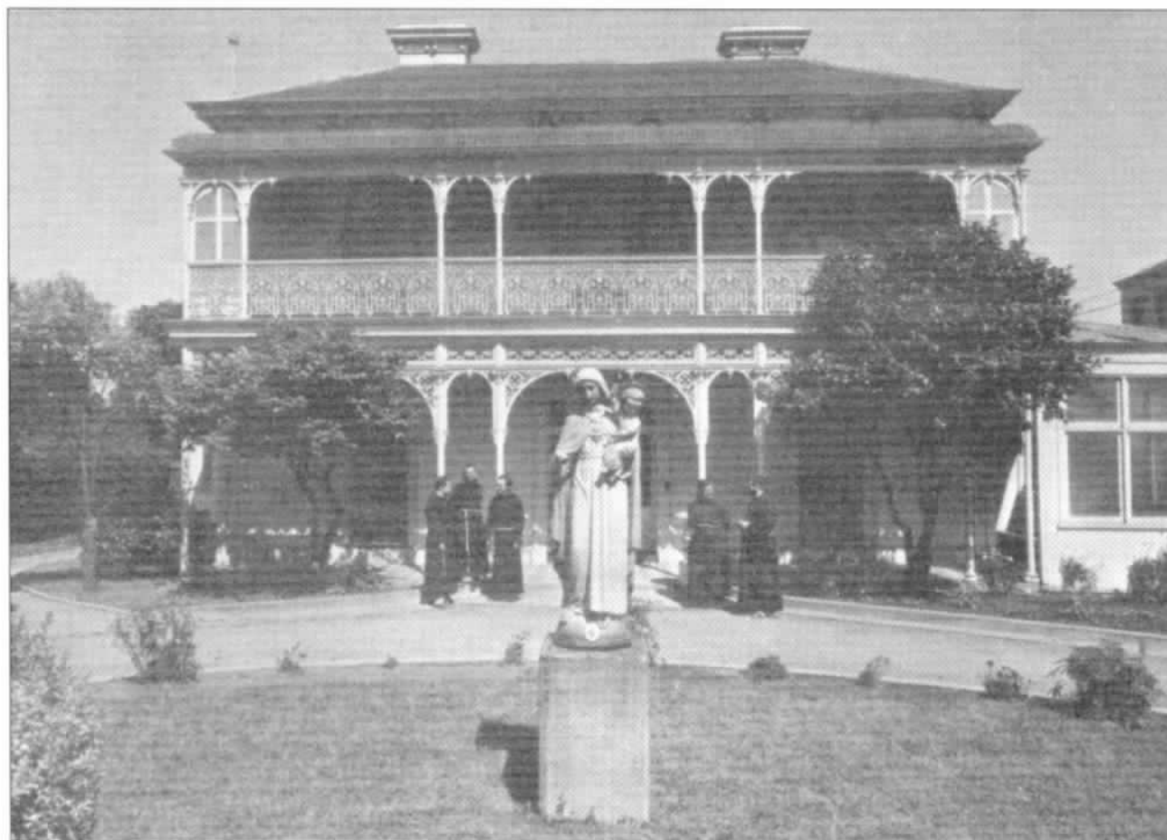
La 'Casa del Sacerdote' at 182 Power Street, Hawthorn.
