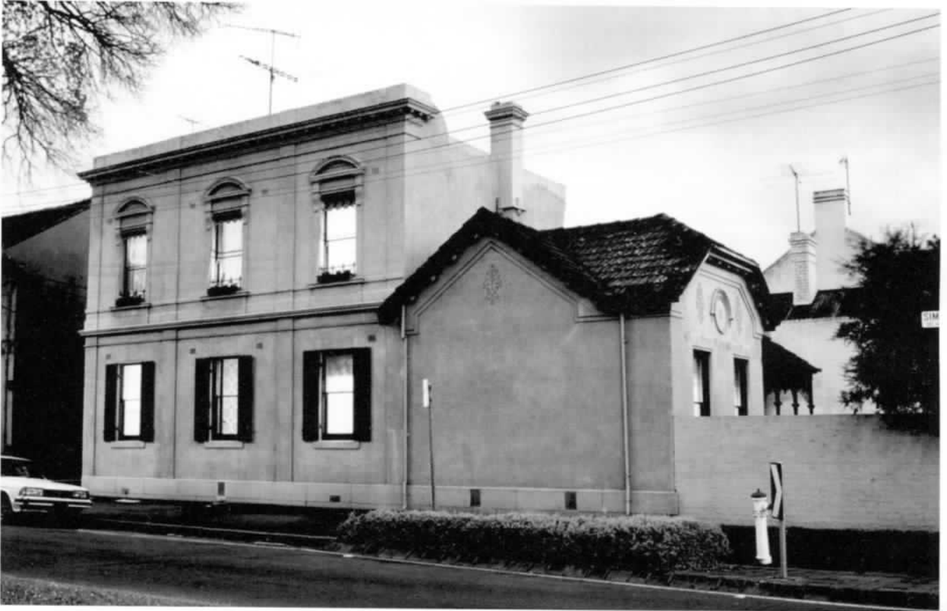
No. 33 Grey Street, East Melbourne, showing the six-roomed two-storey extension designed by Paolo Dattari.
